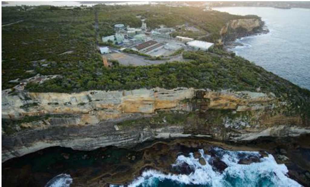
FIGURE 105: NORTH HEAD WASTEWATER TREATMENT PLANT
