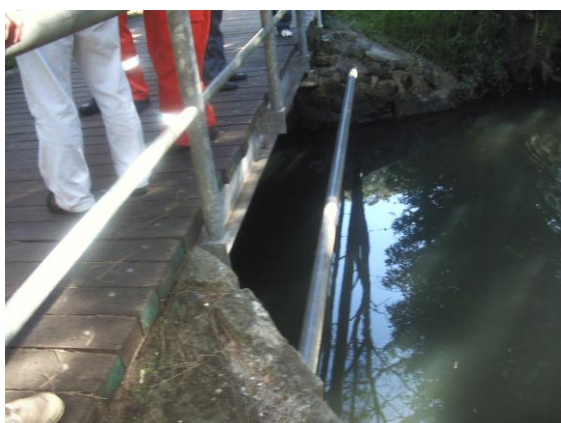
Photo 7: Telstra cable running beneath the 'road bridge' (indicates the original level of the bridge).
