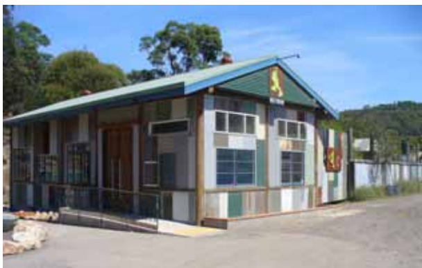
Kimbriki Eco House. Source: Warringah Council
