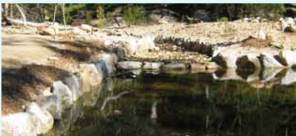
Balmoral Remediation and Creekworks. Source: Mosman Council
