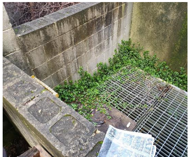
Photo 13: Inlet grate (The Kilns, western channel)
