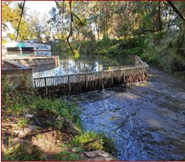
Photo 6: GPT (looking upstream at Harbord Road culverts)
