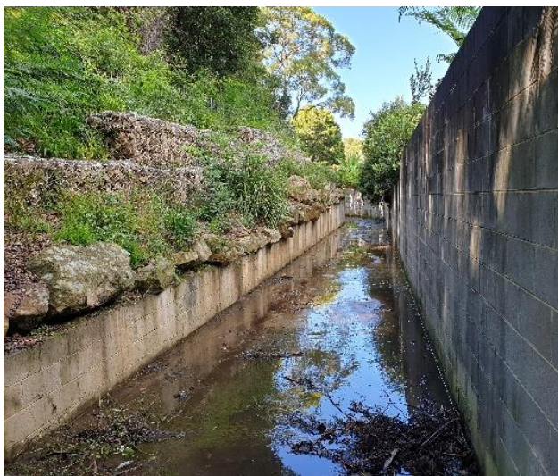
Photo 12: Western stormwater channel at The Kilns (looking downstream)
