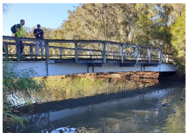
Photo 9: Western pedestrian footbridge (looking upstream)
