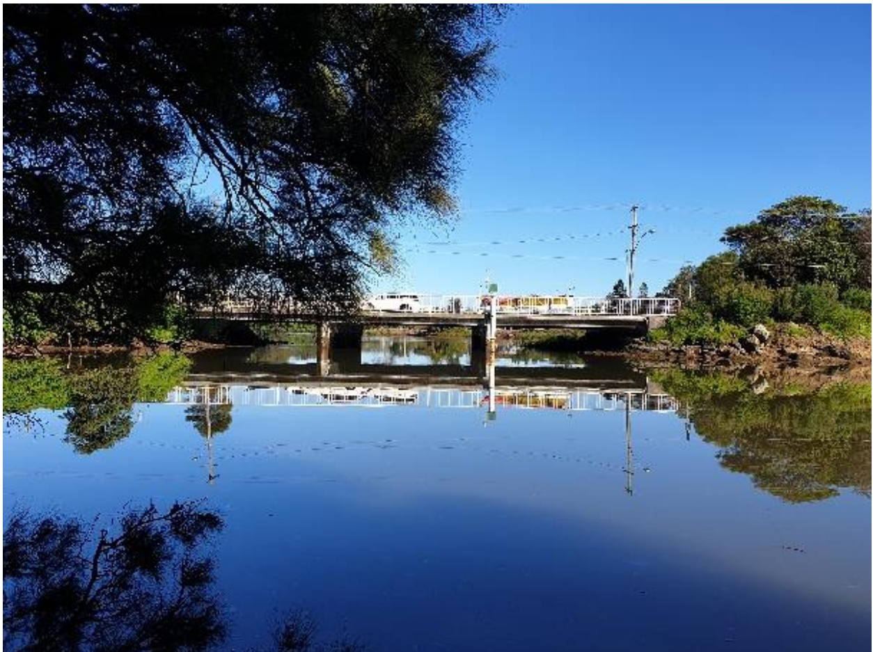
Photo 5: Griffin Road bridge (looking upstream)
