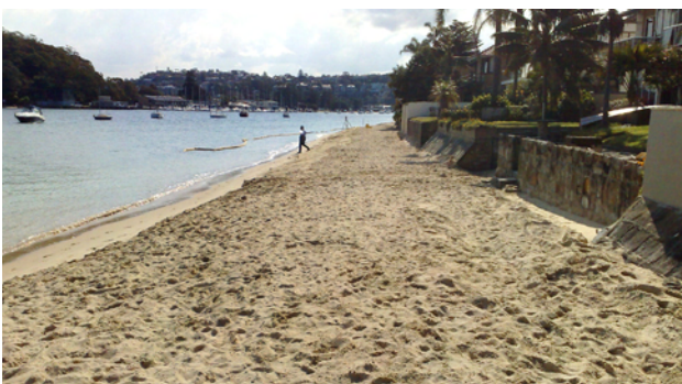
Beach Nourishment at Clontarf. Source: Manly Council.
