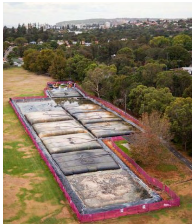
Manly Lagoon Geobag Dewatering Site. Source: Manly Council.
