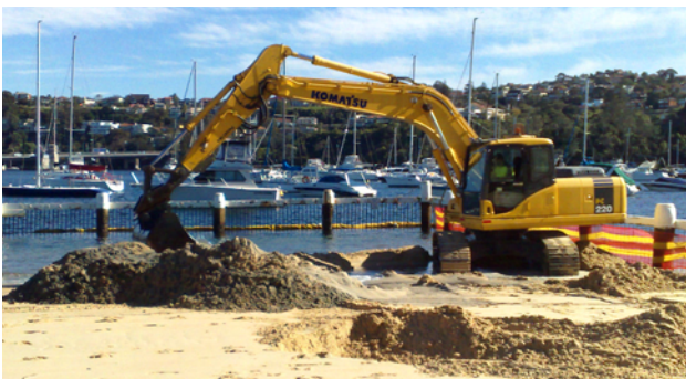
Dredging of Clontarf Swimming Enclosure. Source: Manly Council.
