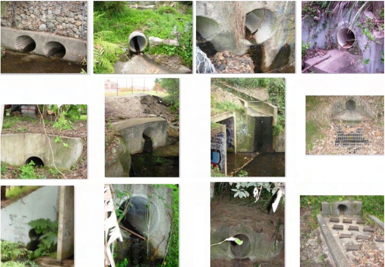
Burnt Bridge Creek Stormwater Drainage Pipes Assessed. Source Manly Council.
