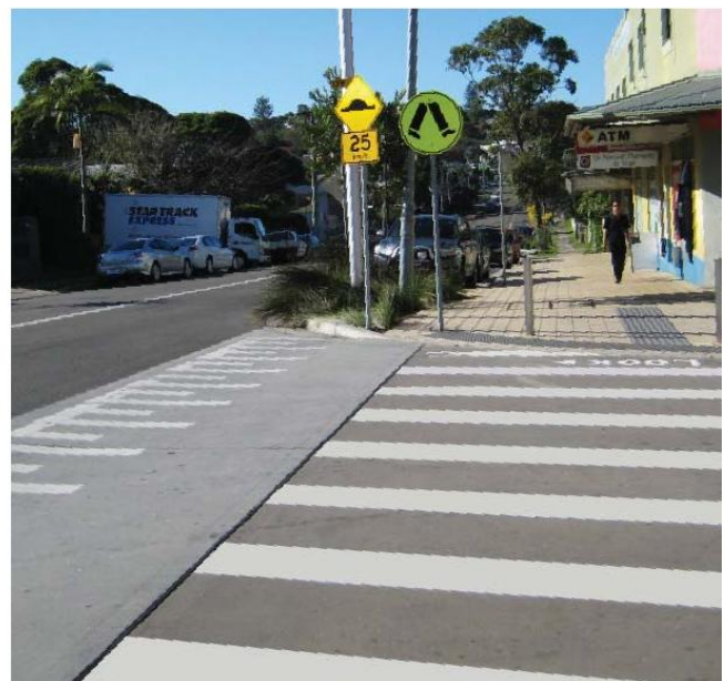
Figure 22: Raised pedestrian crossing, Freshwater
