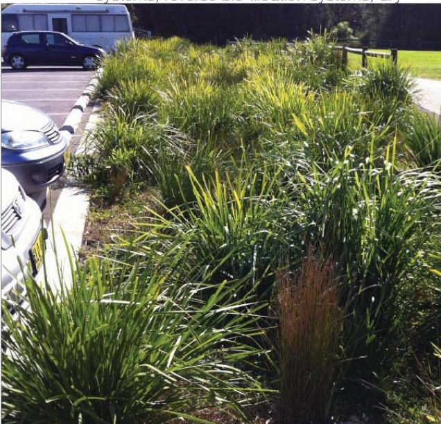
Figure 27: WSUD swale, Richmond Ave Carpark, Dee Why
