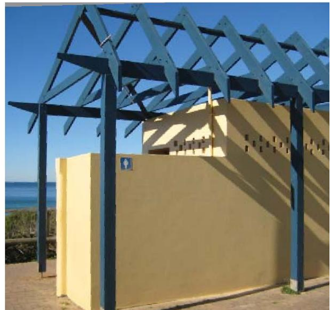
Figure 36: Amenities building, Narrabeen Beach
