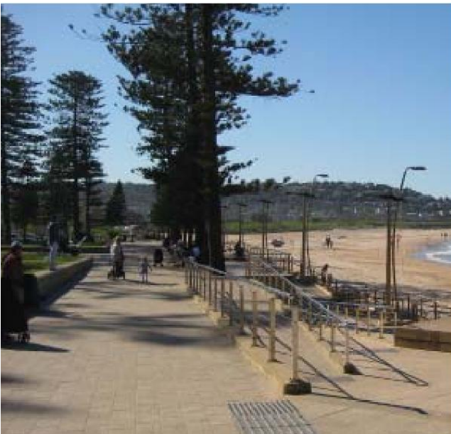
Figure 15: Custom foreshore treatment, Dee Why Beach
