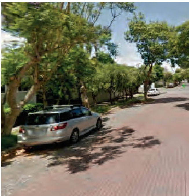
PERMEABLE PAVEMENT AT SMITH STREET MANLY// ASPECT STUDIOS
