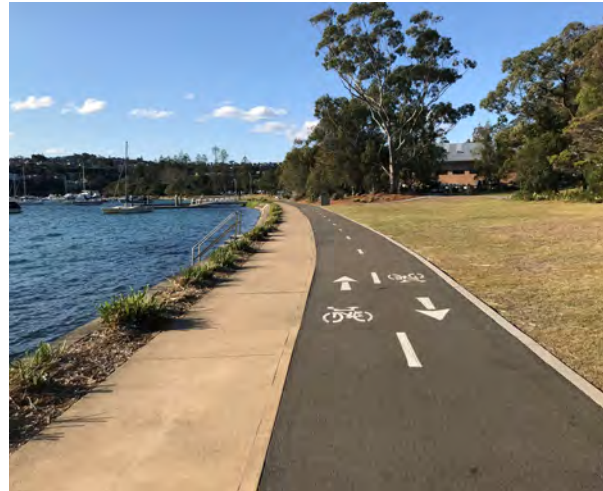
Separated cycleway in park
