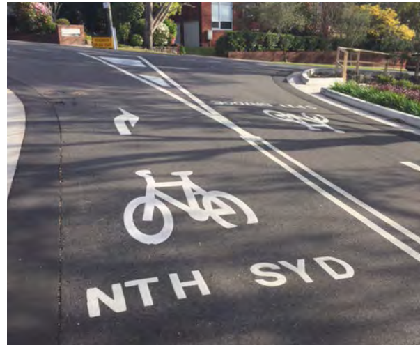
On road directional markings
