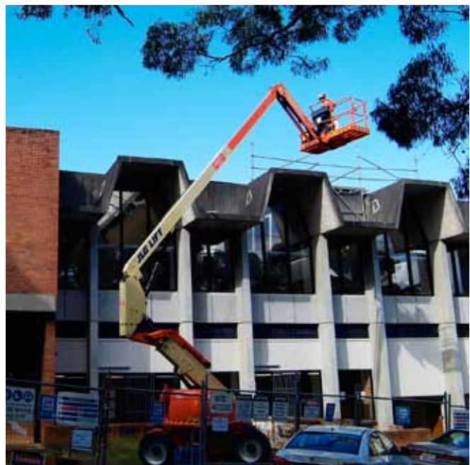
Repairs to the Warringah Aquatic Centre's roof
