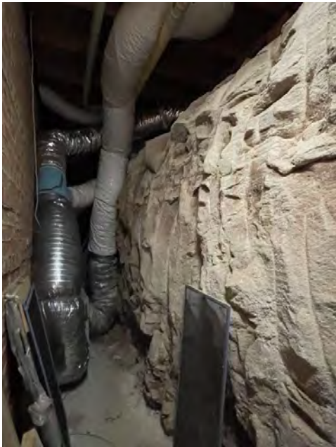
Figure 13 - character of existing rock excavation behind the garage
