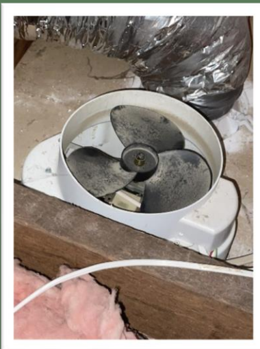
Unsealed exhaust fans & bathroom heating lamps
