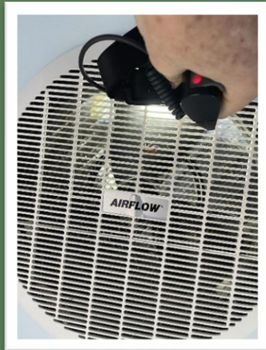
Unsealed exhaust fans & bathroom heating lamps
