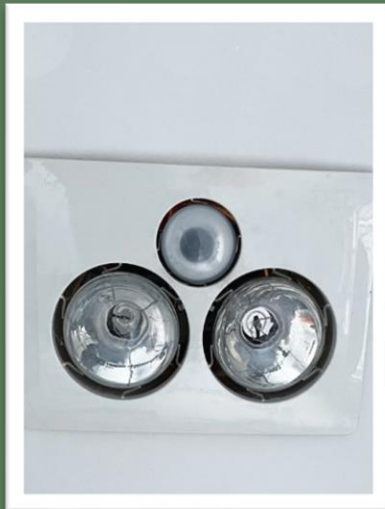
Unsealed exhaust fans & bathroom heating lamps
