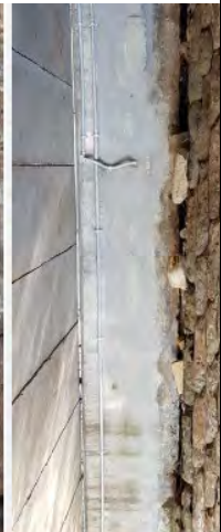
Photo No: 27 Ab Evidence of possible settlement
